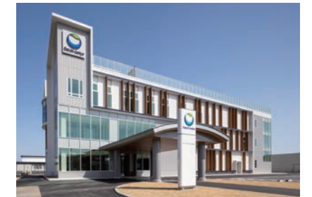
Daiichi Sankyo Chemical Pharma Onahama Plant New management building
