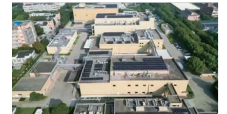
Daiichi Sankyo Pharmaceutical (Shanghai) Shanghai Plant
